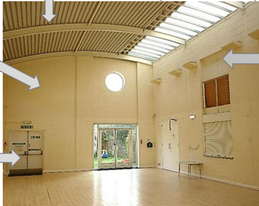
Insulated acoustic lining added to curved metal ceilings
